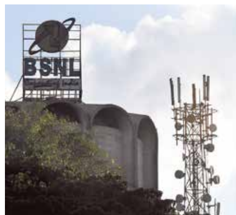
A view of the BSNL building in Bengaluru. ■ 81
